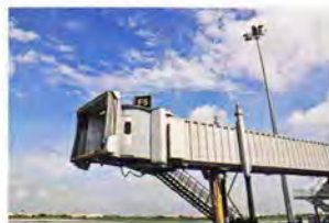
4 Loading Bridge (Jet Bridge)
